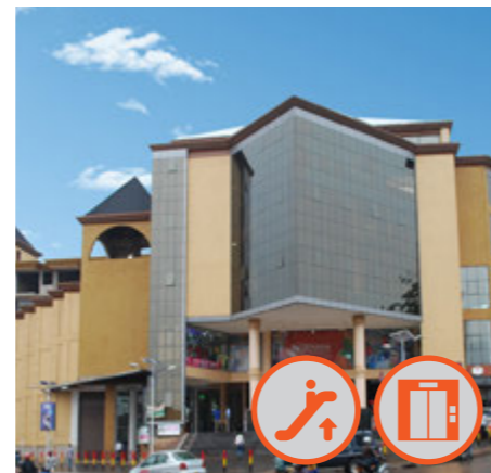
SENANA SHOPPING CENTER Uganda Passenger elevator 4 units, escalator 6 units
