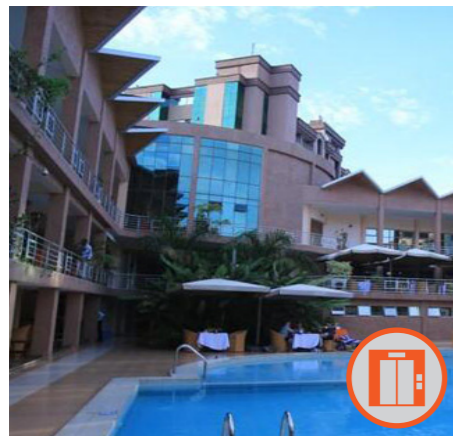
LEMIGO HOTEL Kigali, Rwanda Passenger elevator 6 units
