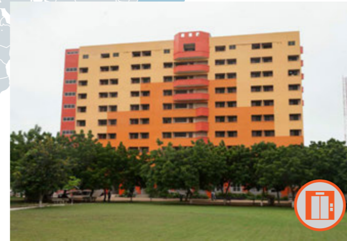
GHANA HOTEL Accra, Ghana Passenger elevator 2 units
