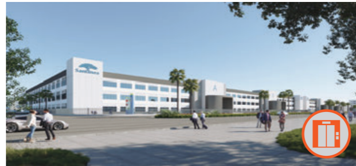
SAMANEA CAMBODIA PHNOM PENH LIGHT INDUSTRY PARK Cambodia Elevator 25 units
