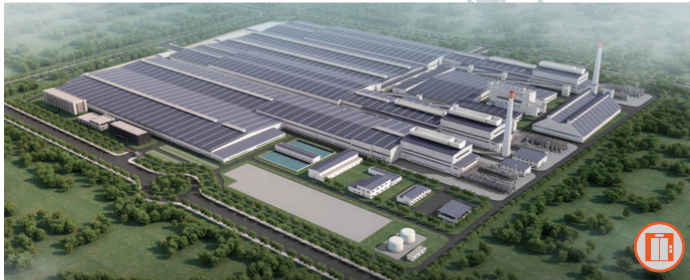
SBH KIBING SOLAR NEW MATERIAL(M) SDN.BHD Malaysia Elevator 12 units (Include CE 18tons)
