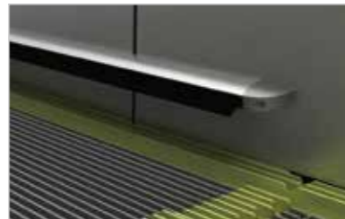
Skirt-panel anti clamp device To prevent passengers from standing too close to the edge of the steps, avoid the steps will pull the foot into the gap between the stairs and the skirt panel.
