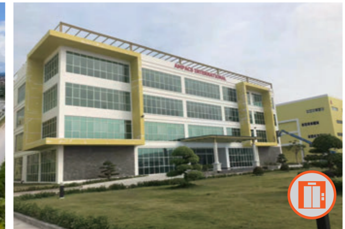
AMPACS INTERNATIONAL Binh Duong, Vietnam Passenger Elevator 1 units Freight Elevator 13 units
