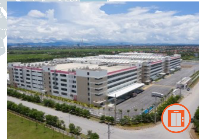
REGINA MIRACLE INTERNATIONAL (VIETNAM) LIMITED Haiphong, Vietnam Passenger Elevator 14 units Freight Elevator 33 units
