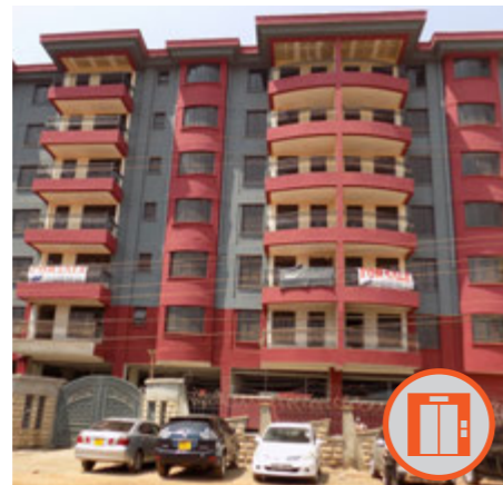
DAINTY APARTMENT Nairobi, Kenya Passenger elevator 2 units
