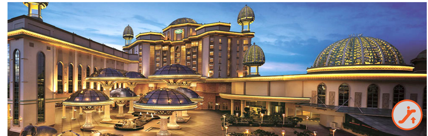
SUNWAY GROUP PROJECT Kuala Lumpur, Malaysia Escalator 8 units
